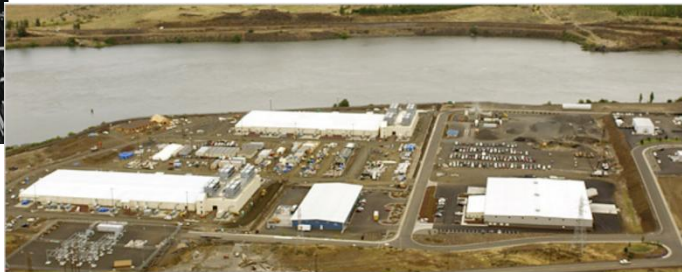
Data Center, Oregon →
